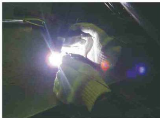
The unique technique on Tungsten inert Gas welder.
