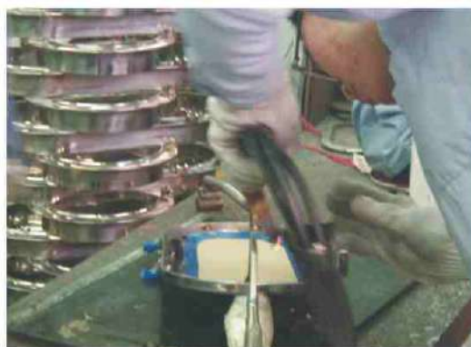
Expert craftsmen are proceeding the welding.
